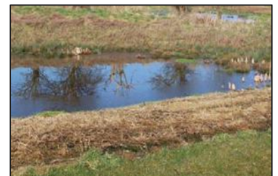
An attenuation basin, as well as allowing safe and contained storage for excess rain and storm water, could deliver opportunities for further biodiversity net gain.
